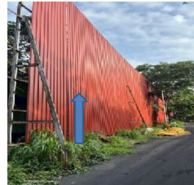
12mtr barricade to prevent fly of dust particles (At RPC unloading Area)
