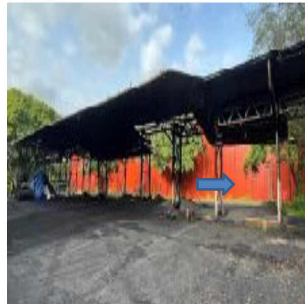
12mtr barricade to prevent fly of dust particles (At RPC unloading Area)
